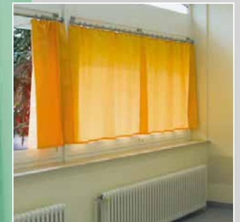
Mounting above the lintel
